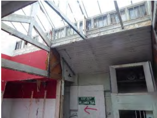
Figure 37 Boarded soffits in parallel range to south
